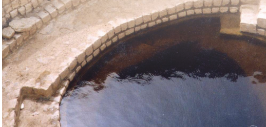
Yemen: Restoration of traditional cisterns
