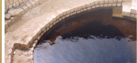
Yemen: Restoration of traditional cisterns
