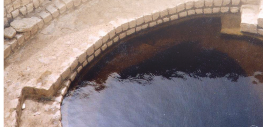
Yemen: Restoration of traditional cisterns
